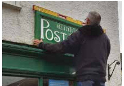
Robert Baker putting the repaired sign up
